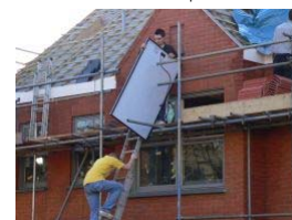
Solar panel going up
